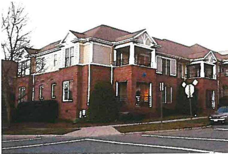
Figure 6-7-10: Heavier materials below lighter elements
